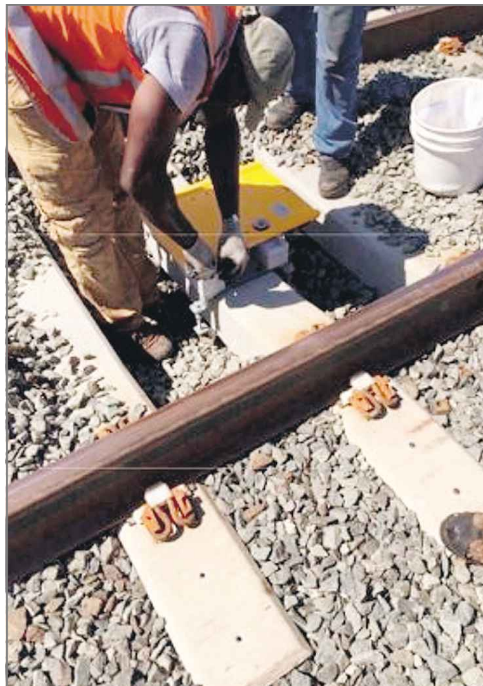
Workers install a radio transponder for positive train control on an LIRR track. The transponders communicate to stop speeding trains.
